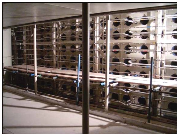
Nozzle Array Erection at Taweelah B Plant
