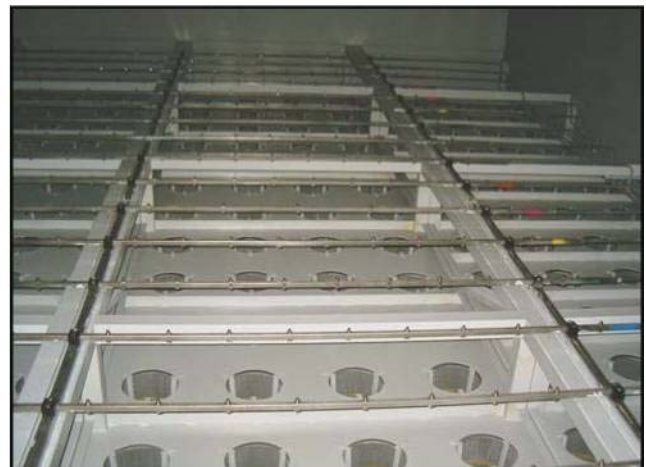
Air Intake Nozzle Array Installation at Escatron
