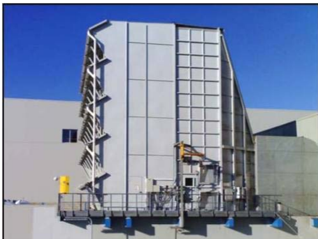
Air Intake Nozzle Array Installation at Escatron
